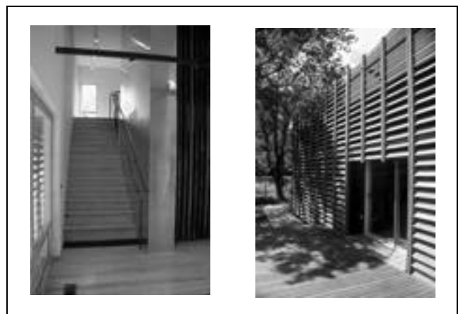
Two views of 1603 Random Road: Interior Stairway and Exterior Louvered Siding on South Side.
